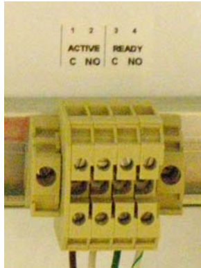
Figure 3-2: Control Connections at TS1
