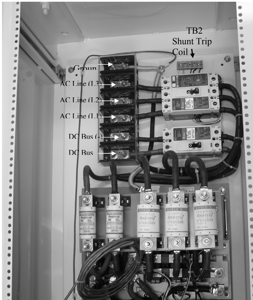
Figure 3-5: F39 Cabinet Field Connections
