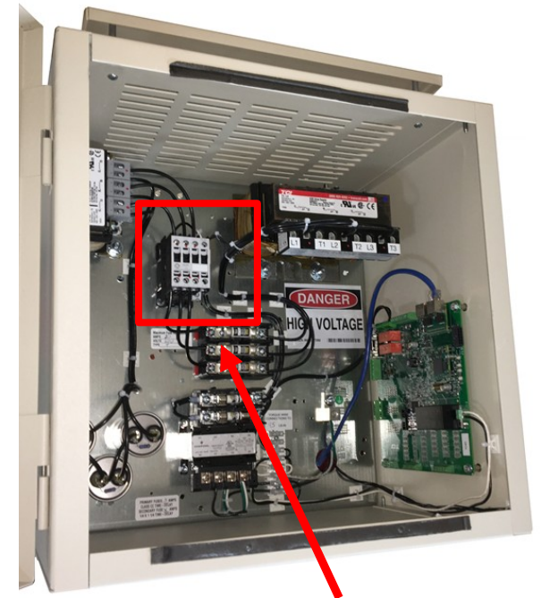
25HP HGP with Isolation Contactor
